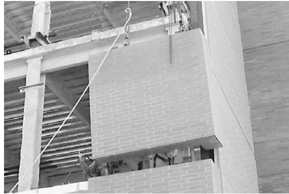
Figure 15-59 Lifting a prefabricated masonry panel into place.
